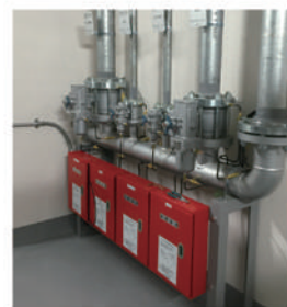
Selection Valve / Manifold Pipe / Pilot Cylinder Unit
