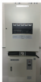
Control Panel / Emergency Power Supply Unit
