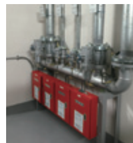
Selection Valve / Manifold Pipe / Pilot Cylinder Unit
